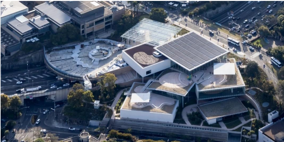
Figure 2 – New building Naala Badu, with land bridge over Eastern Distributor motorway (running top right to bottom left), and original building Naala Nura top left (© Iwan Baan)
