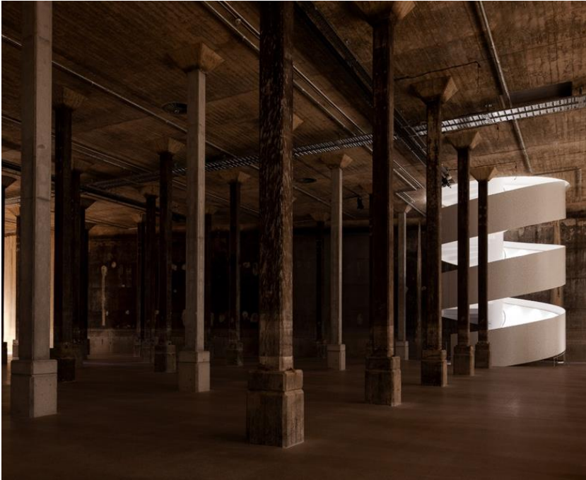
Figure 7 – New columns (lighter grey) among original columns, with new stair. (© Iwan Baan)
