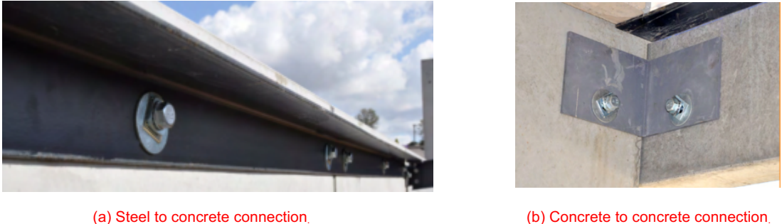
Figure 1. Typical Bolted/cast-in connections
