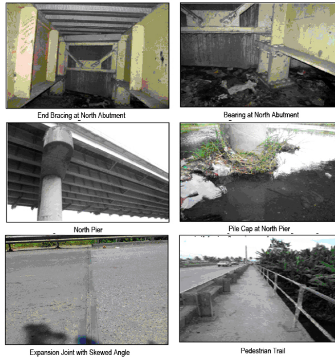
Figure 10: Photos of Butibam Bridge
