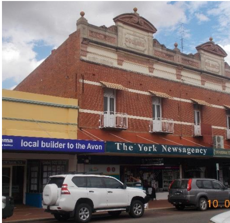
(a) Parapet front view
