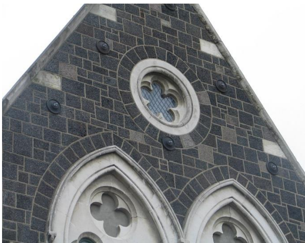
(a) Gable wall ties to roof structure
