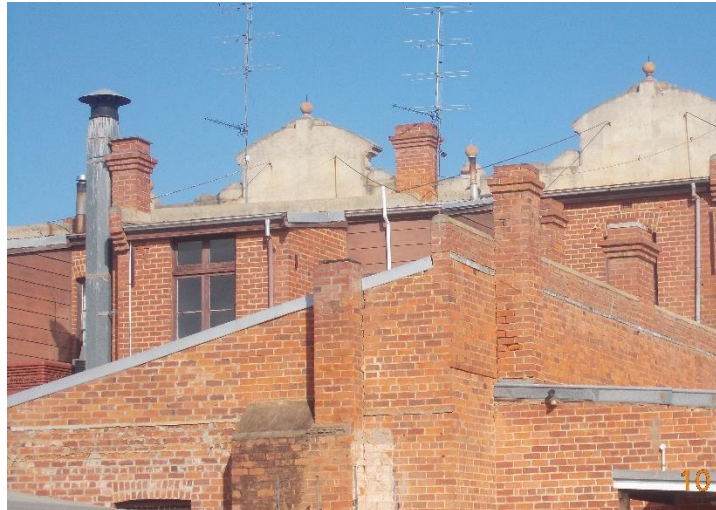
(b) Rear view, note point connection for parapet restraint
