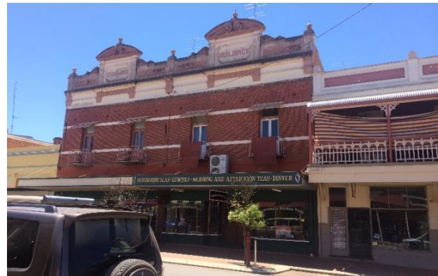
Figure 2. Example of a two storey retail URM building in York.
