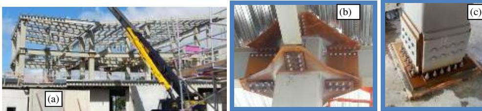
Figure 7. Details of the Friction Connections on the Terrace Project (MacRae)
