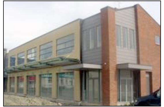
(c) New south and east walls, after redevelopment
