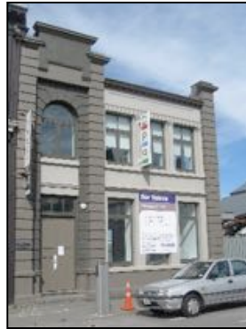
(b) West façade, after retrofit
