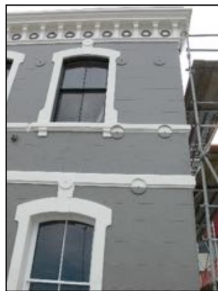
(f) Wall anchors painted to match façade, 2011
