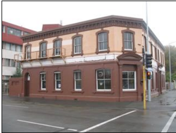
(a) Before retrofit, June 2010
