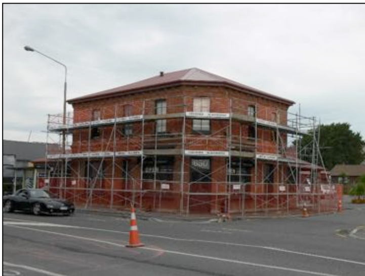
(e) Exterior repairs underway after 22 February 2011
