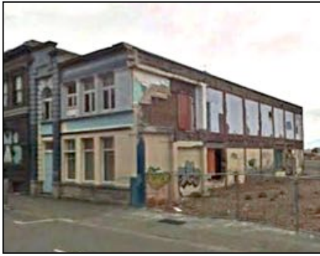
(a) Façade and south wall, before retrofit
