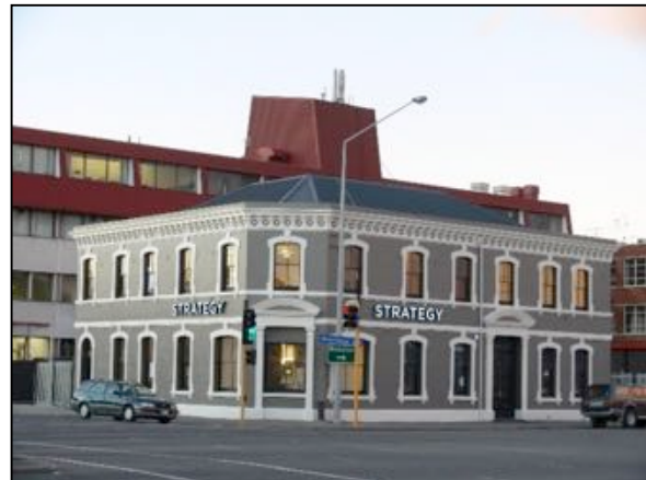
(b) After retrofit, September 2011
