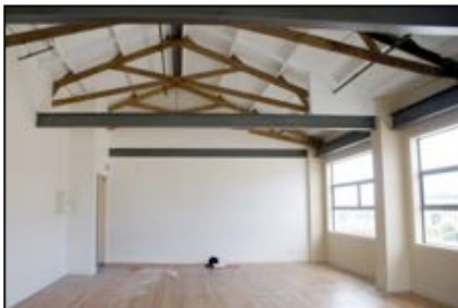
(e) First floor interior looking east, after retrofit
