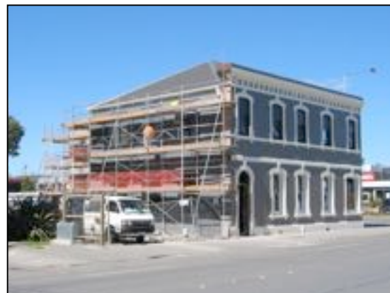
(g) Undamaged building, days after the 22 February 2011 earthquake.
