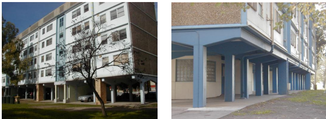
Figure 1. Category 1 building with soft- and/or weak-storey in Melbourne.
