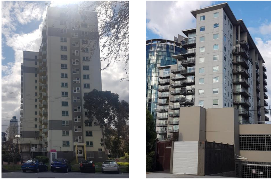
Figure 3. Category 2 building with perimeter RC walls.
