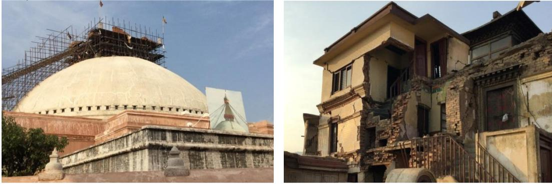
Figure 2. Damaged structures of (left) the Boudha Stupa in the eastern Kathmandu Valley and (right) a house near Swayambhunath Stupa in the western Kathmandu Valley (photographs were taken in April, 2016, one year after the Gorkha Earthquake).
