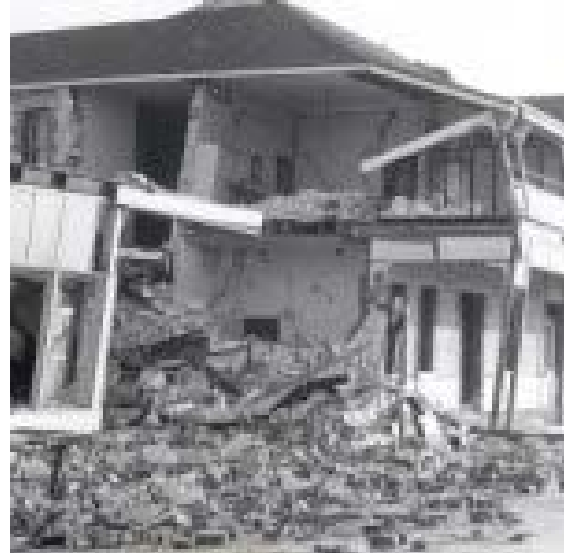
Figure 4: The damage to the Meckering hotel. Photograph courtesy of AEES.
