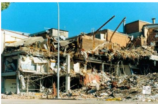
Figure 8: Collapse of Workers Club. Photograph courtesy Newcastle Council Earthquake Collection, Newcastle Region Library Ref No. 046 000 544.
