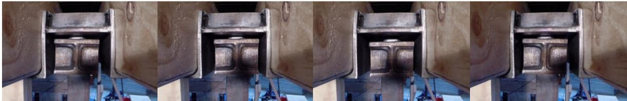
Figure 5 - Gap between corbel and inside of saddle bracket to accommodate bidirectional movement
