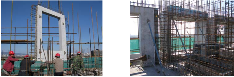
Fig.1 Precast panels utilized in apartment building
