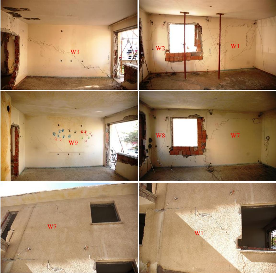
**Fig. 9 – Observed wall damages**
