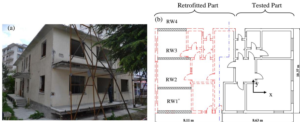
**Fig. 1 – Test structure : (a) Photo and (b) Plan view of tested masonry structure (\*: Retrofitted Wall)**
