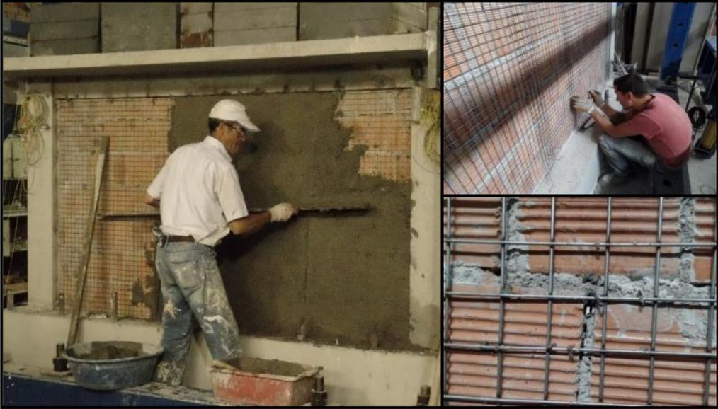
Fig 4. Construction details of SMF
