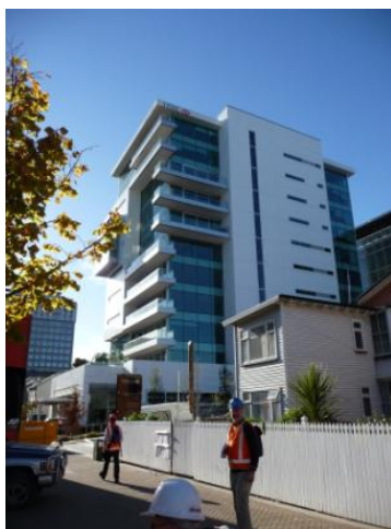
(a) Overall view of tower from North West Corner [M Bruneau]
