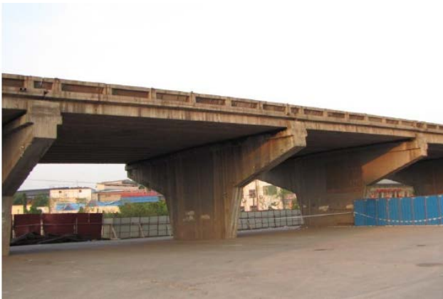
Fig.1. Typical view of Hongqi Viaduct (before collapse).
