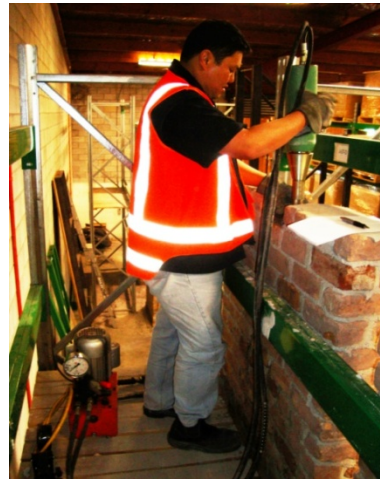
(b) Posttensioning of PTS-02
