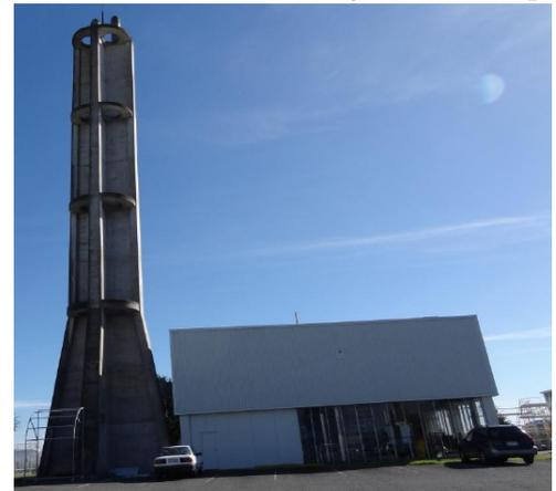
Figure 1. Rocking chimney at Christchurch airport (car for scale).
