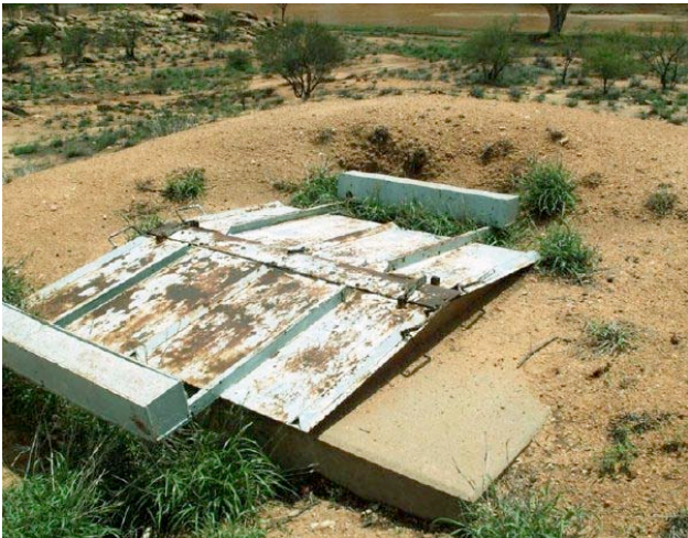
The entrance to the vault at the base of Spencer Hill near Alice Springs showing the counterbalanced steel doors atop a steel-lined vertical shaft.
