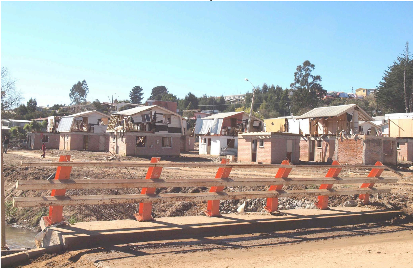
Tsunami damage Dichato, Chile (photo Gary Gibson)
