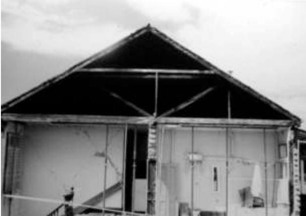
**Photo 3 Building damage, lack of connectivity**
