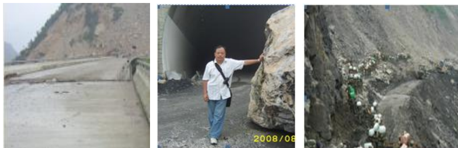
(a) Tunnel entrance is covered by rock landslide (b, c) traffic is blocked by falling rocks
