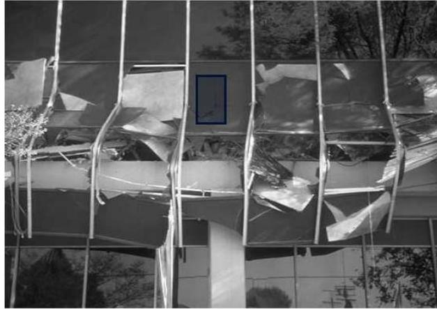
*Figure 1 Kaiser Permanente Building, Granada Hills, California, cladding offset NISEE Steinbruggecollection, photo by Mark Aschheim), (Shahram and Miranda 2003)*
