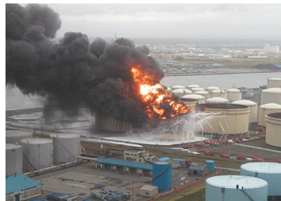
Whole surface fire of tank
