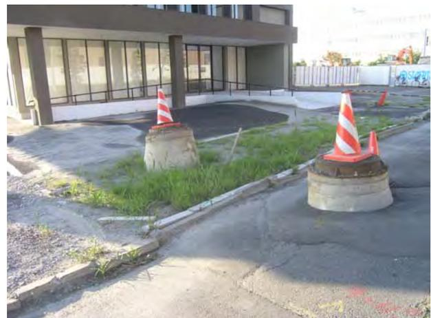
Fig. 20 Floating of a series of manholes
