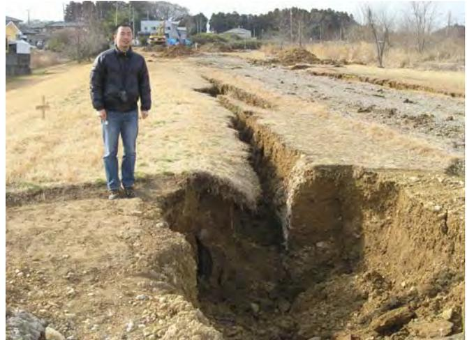
Fig. 12 Liquefaction-induced lateral spread and subsidence of Naka River levee
