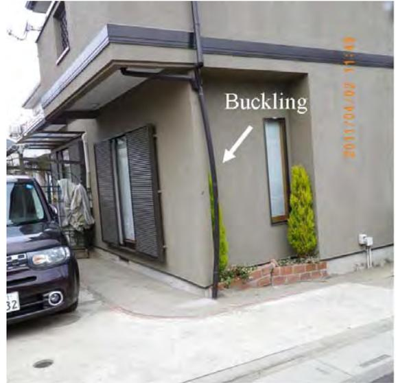
Fig. 29 Liquefaction-induced tilting (Kazo City)
