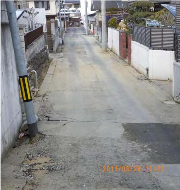
Fig. 10 Remains of liquefied sand at road surface in residential area where former water stream was filled with cut soil
