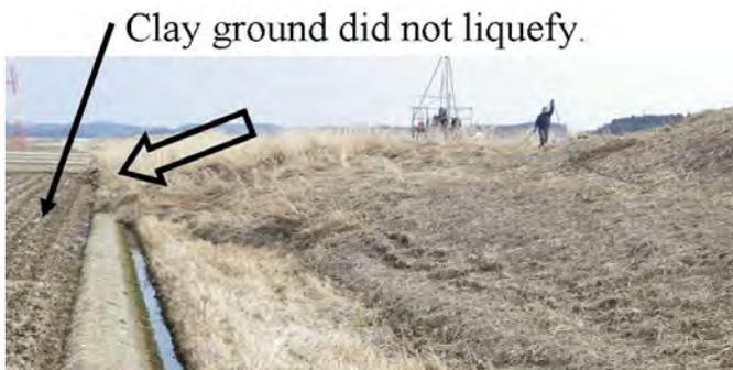
Fig. 14 Damaged levee resting on unliquefiable clayey subsoil (levee of Naruse River, north of Sendai)
