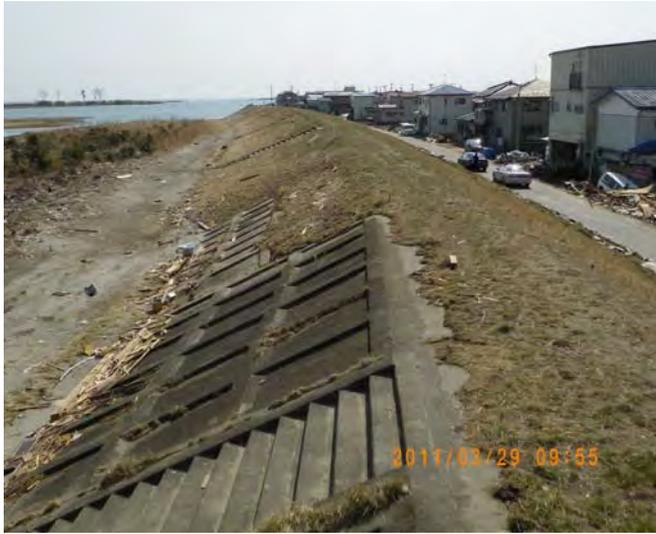
Fig. 6 River levee that survived tsunami in spite of overtopping (Natori River at Yuriage)
