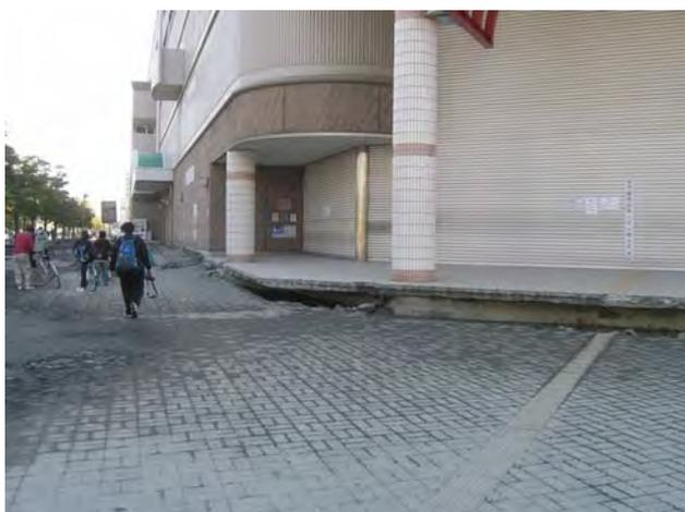
Fig. 18 Differential settlement between surface of liquefied ground and pile-supported building
