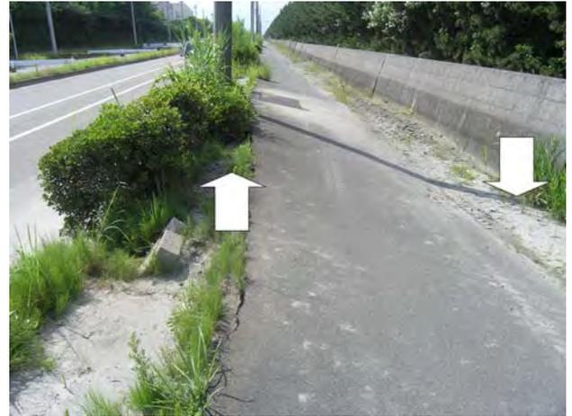
Fig. 23 Liquefaction-induced distortion of sidewalk
