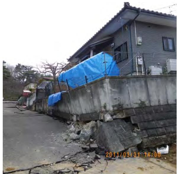
Fig. 9 Damaged residential fill in Sendai
