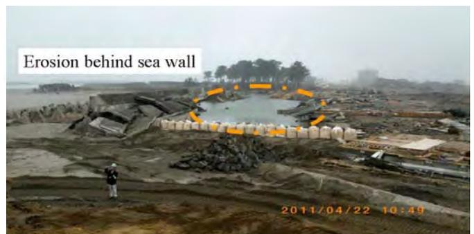
Fig. 5 Destroyed shape of sea wall (near the mouth of Abukuma River to the south of Sendai City)
