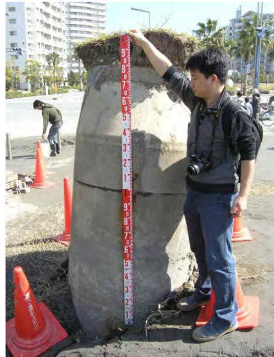
Fig. 19 2-meter floating of manhole
