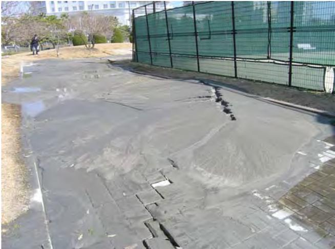
Fig. 16 Liquefaction and sand ejection in Urayasu City
