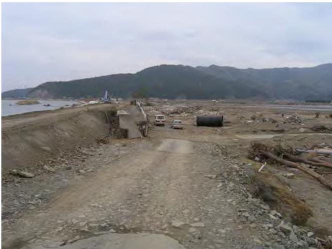
Fig. 7 Damage of Kitakami River levee that was directly hit by tsunami
