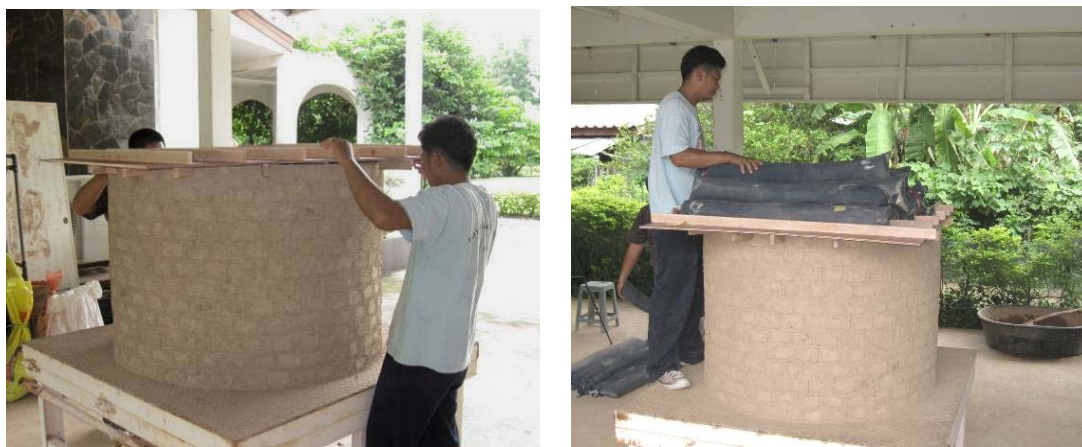
Figure 2: Roof and sand bags installation.
