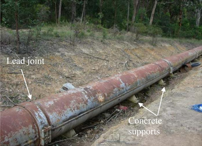
Figure 2: A photo of the pipeline showing the lead joints and concrete supports.
