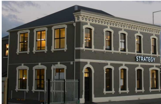
Figure 7 - Successfully retrofitted Christchurch URM building (May 2011)
