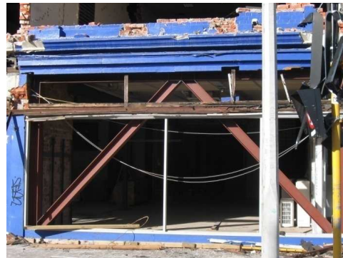
b) URM building with visible retrofit
