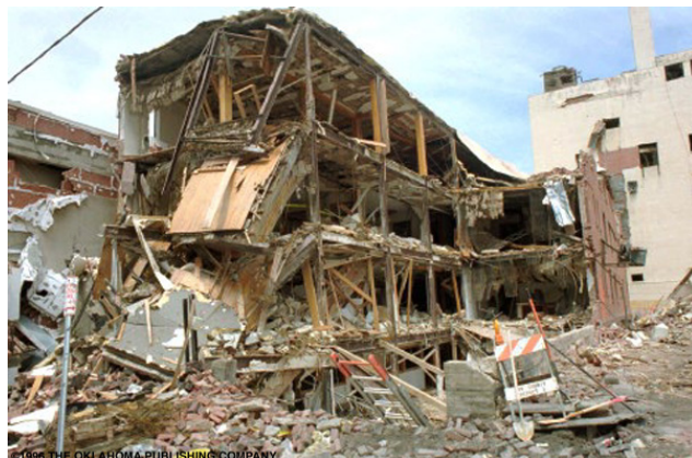
Figure 3: Disproportionate collapse — Oklahoma 1995
