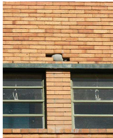
Figure 4: Bricks removed to demonstrate expanded grout sock
