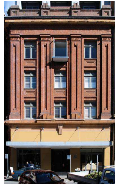
Figure 1: Typical undamaged building in Newcastle
