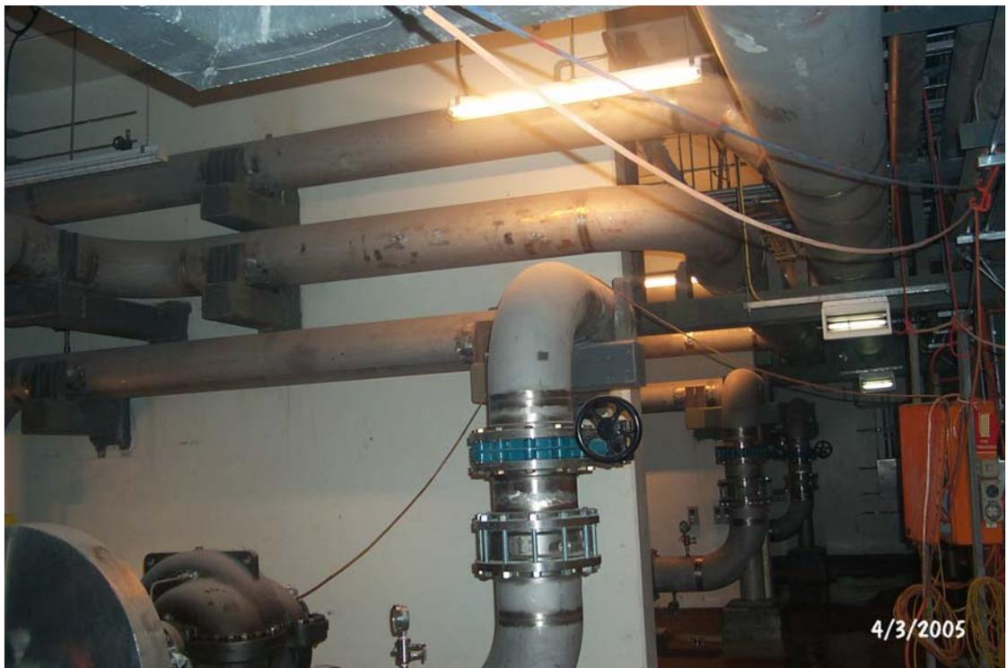
**Figure 2 --OPAL Seismic Supports for Primary Circuit Piping**
