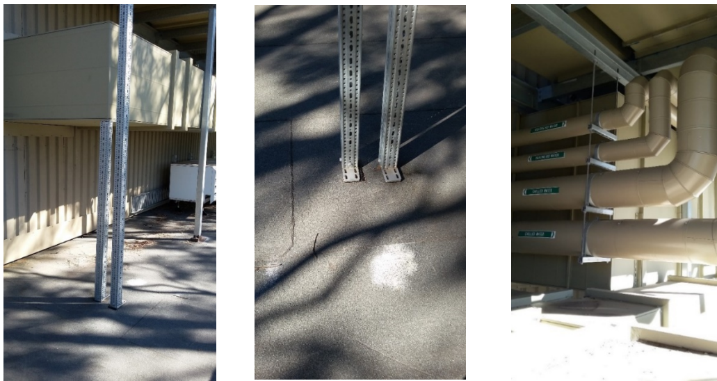
Figure 6: Duct Supports without any positive connection to roof (without base plate) and gravity pipes without any seismic restraints 2018 Governmental building Sydney
