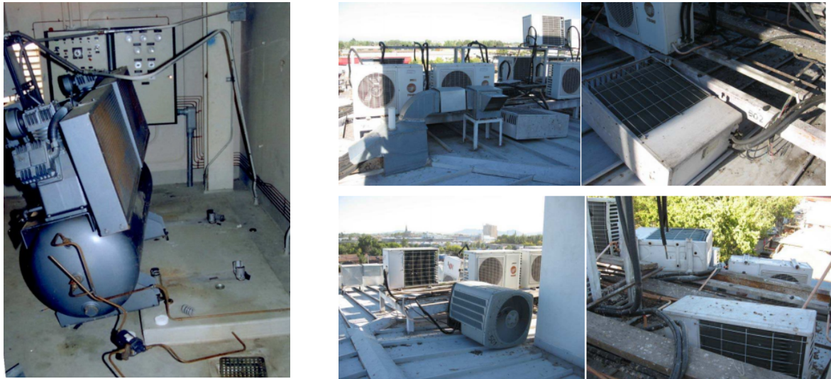
Figure 2: Compressor failure in 1994 Northridge and Rooftop condensing units toppled in 2010 Chile
