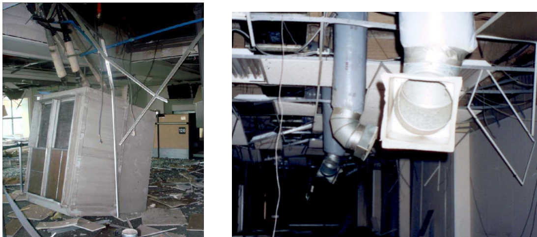
Figure 3: HVAC equipment failure in 2010 Chile and Air diffusers collapse 1994 Northridge
