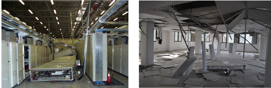
Figure 5: Electrical Cabinets overturned 1999 Izmit and Lighting dangling 2010 Haiti
