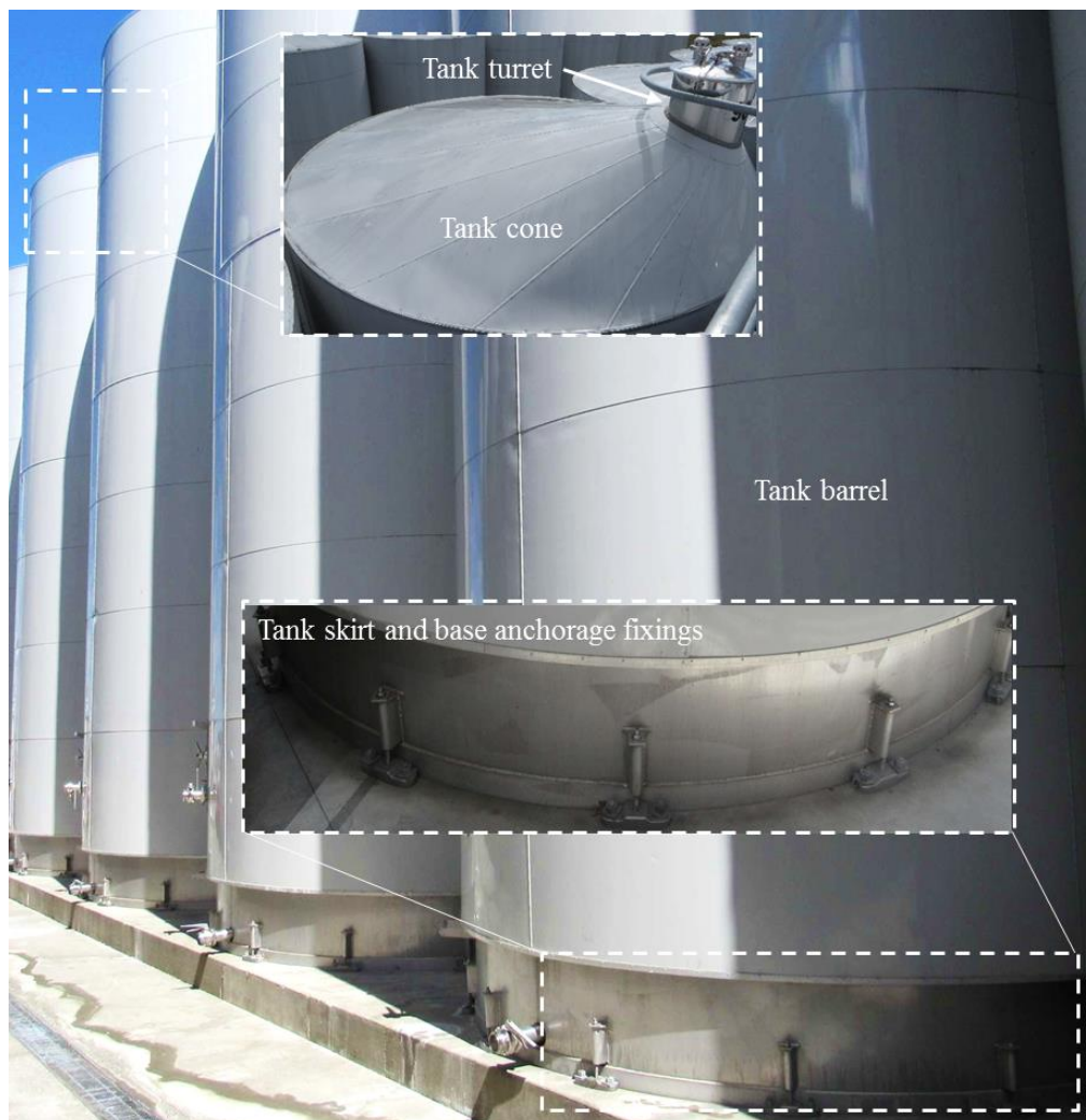
Figure 1. Different parts of typical flat-based wine tanks
