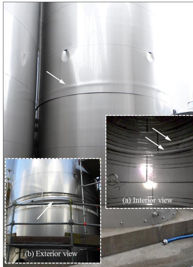
Figure 6. The case study tank (240 kL) showing elephant-foot buckling (indicated with arrows) following the 2016 Kaikōura earthquake. (a) Interior view of the tanks showing elephant-foot buckling, (b) Exterior view showing the extent of buckling when the external insulation layer was removed.
