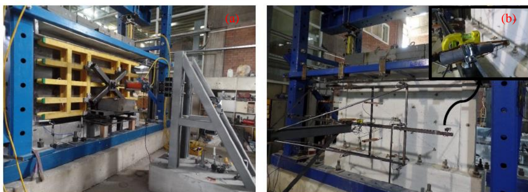
Fig. 4. Test setup and instrumentation for OOP loading: (a) loading setup for airbag and (b) displacement measurements
