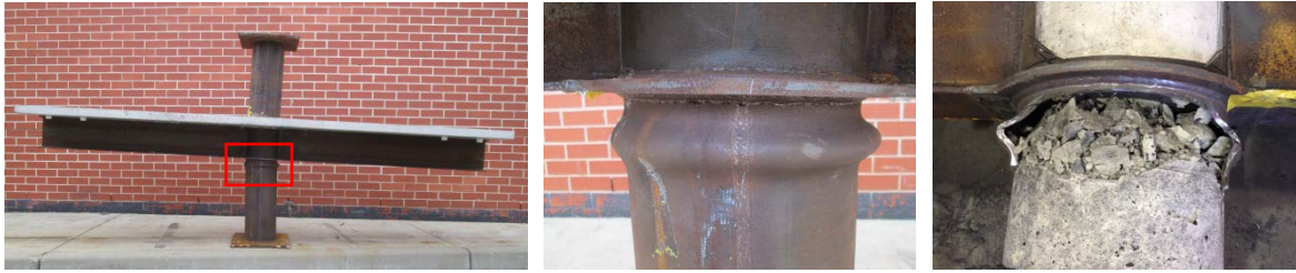
Figure 8. Failure modes of specimen CS-1.
