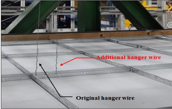
Figure 8. Detachment of the main runner joint Figure 9. Installation of the additional hanger wire
