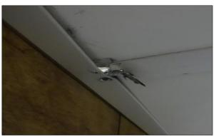
Figure 13. Failure of perimeter connection
