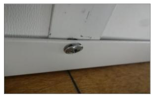
Figure 10. Dislodged tapping screw
