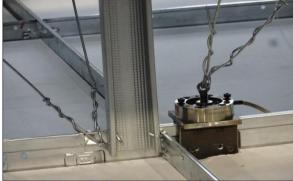
Figure 6. Hanger wires and connection devices
