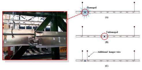
Figure 16. Damage to the connection joint of the main runner
