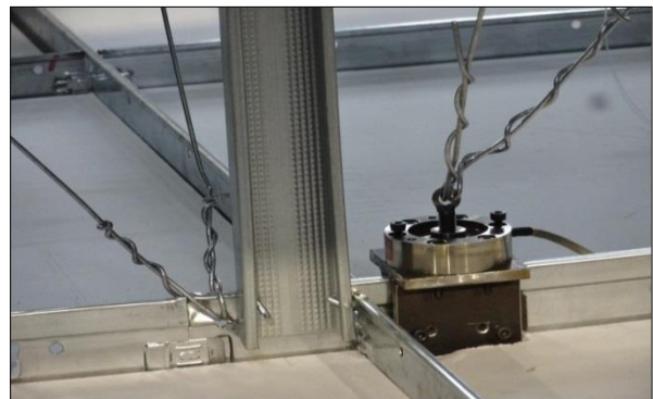
Figure 7. Installation of the load cell
