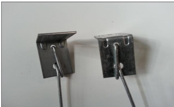
Figure 6. Hanger wires and connection devices
