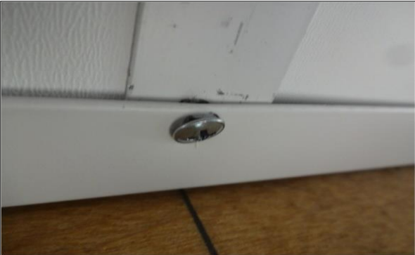
Figure 10. Dislodged tapping screw
