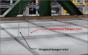
Figure 8. Detachment of the main runner joint
