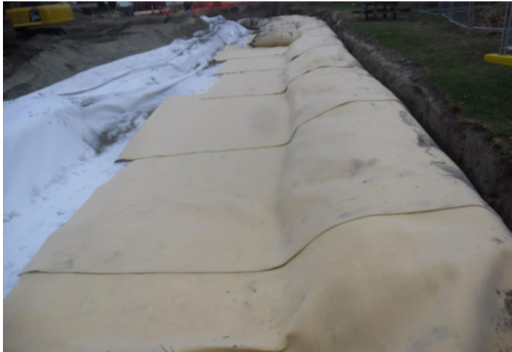
Figure 5 – Alternative system to 0.75m 3 self-healing toe
