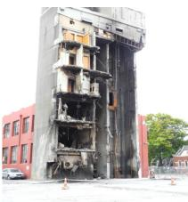
Figure 4: Failure of connection between diaphragm and core, CTV building, Christchurch
