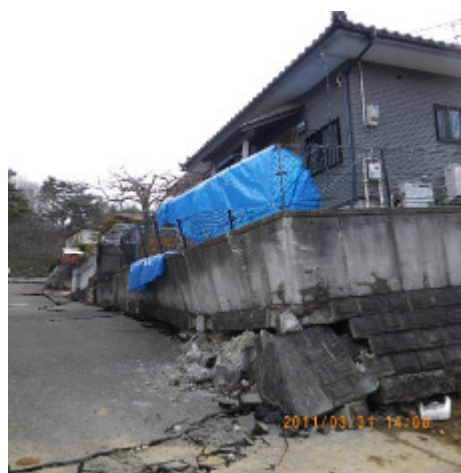
Figure 11 Earthquake damage in a filled part of residential development in hilly area (Oritate of Sendai City)
