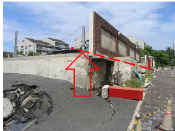
Figure 3 Floating of underground car parking
