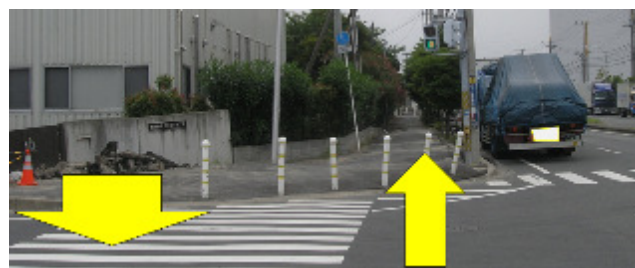
Figure 4 Subsidence of private building into liquefied subsoil induced distortion of public sidewalk
