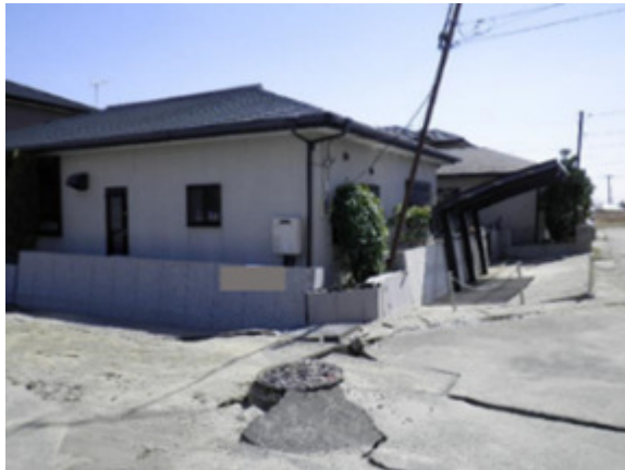
Figure 2 Liquefaction-induced subsidence
