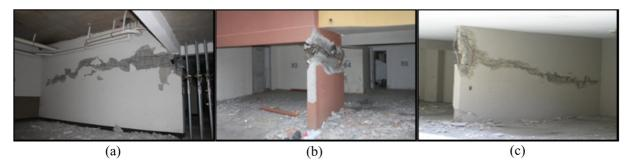
Figure 2. Typical brittle failure in RC walls during the 2010, Maule earthquake: (a) building in Santiago; (b) building in Concepción; and (c) building in Viña del Mar.
