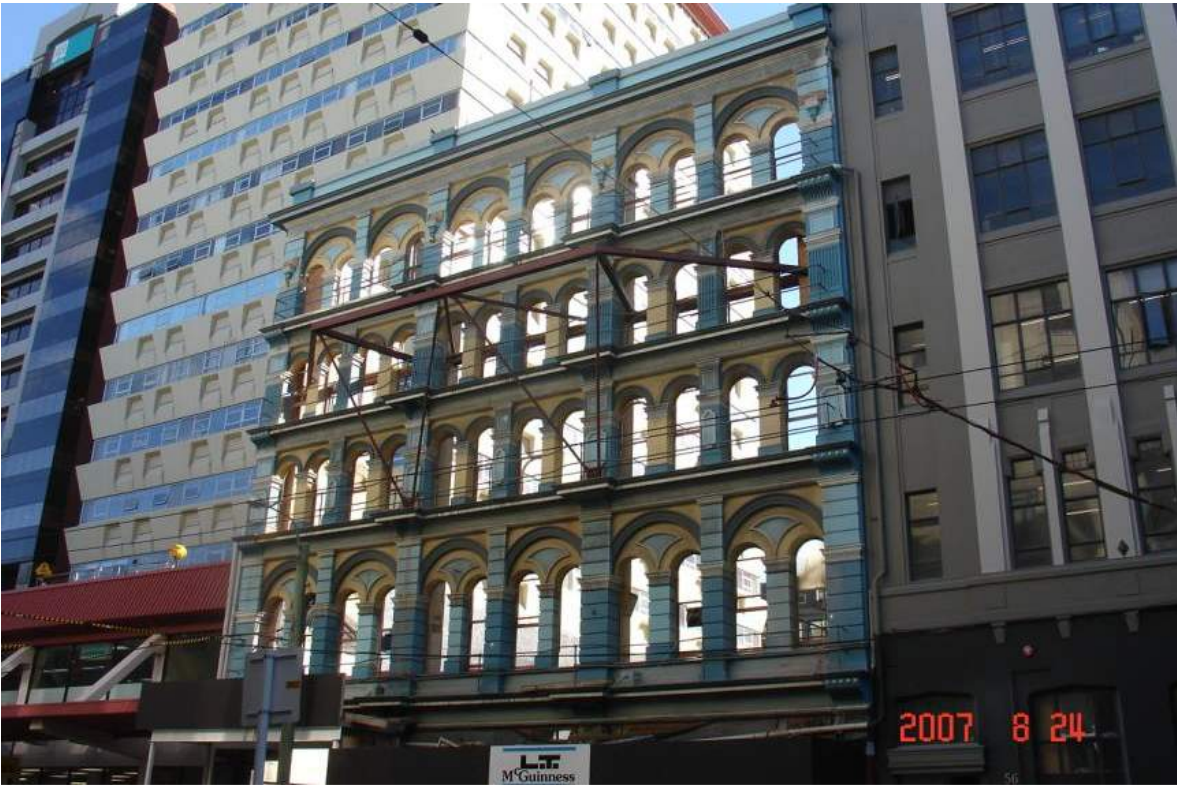
Figure 11: Ballinger Building with temporary facade retention
