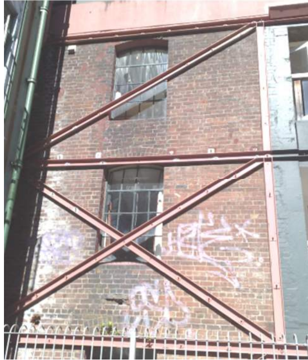
Figure 3: Stiffness incompatibility between strengthening and existing elements
