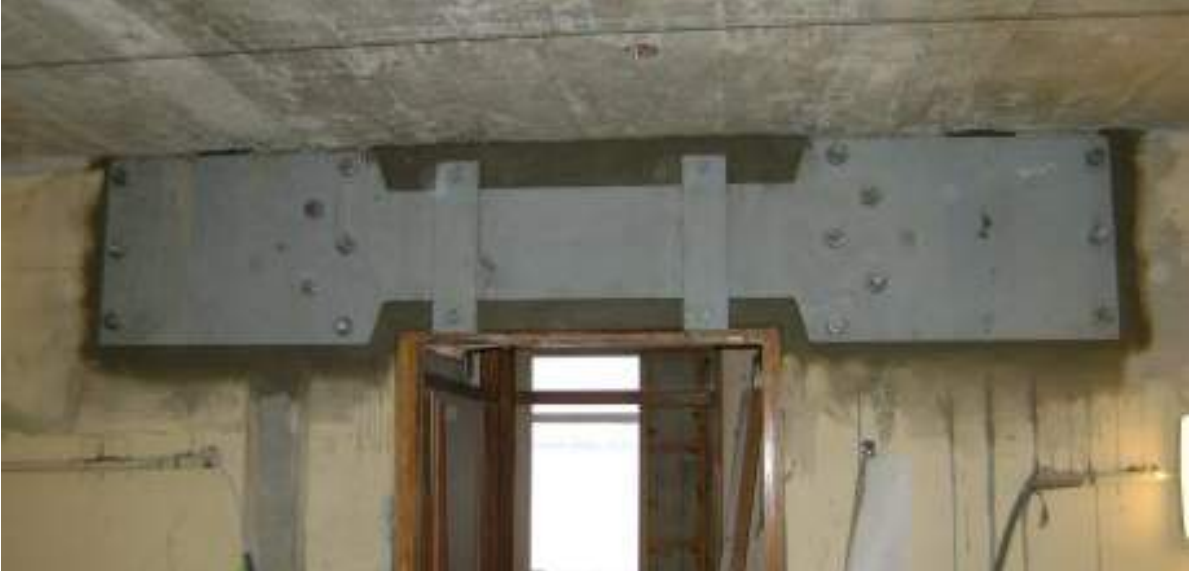
Figure 8: Steel plates forming coupling beams between walls over the existing doorways.
