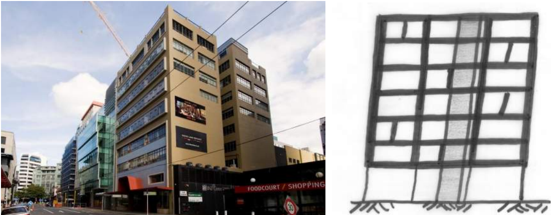
Figure 10: National Mutual building, and illustration of the "Pagoda Column" concept
