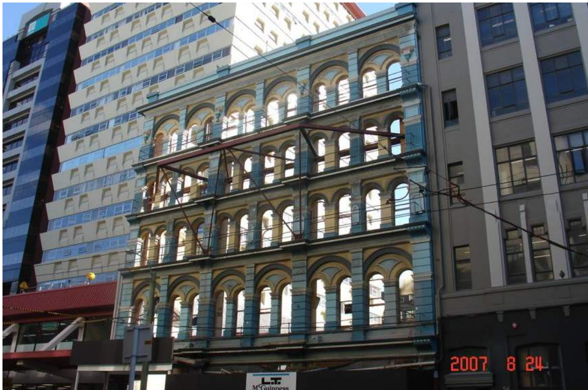
Figure 11: Ballinger Building with temporary facade retention
