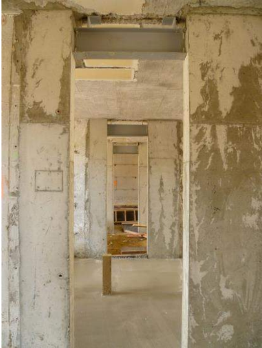
9: New ductile seismic "slots" allowing additional damping and Architectural flexibility.
