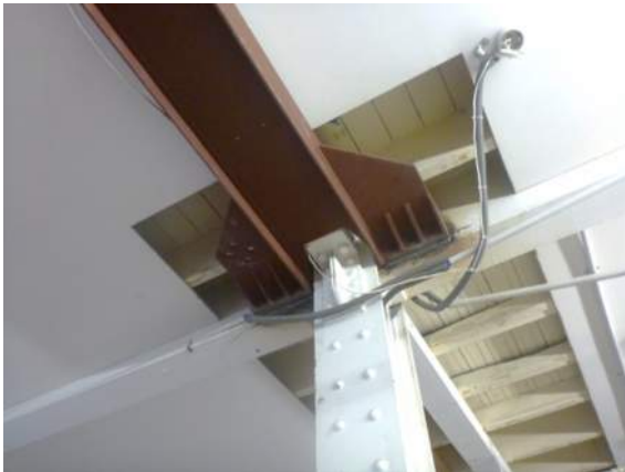
Figure 7: The Woolstore's masonry facade, and examples of the new steelwork detailing
