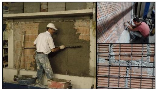
Fig 4. Construction details of SMF
