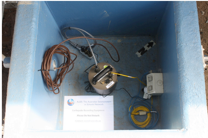
Figure 3. Installation of Guralp CMG-6TD at Ayr State High School, QLD. The seismic vault was made as part of a project by the schools construction class.
