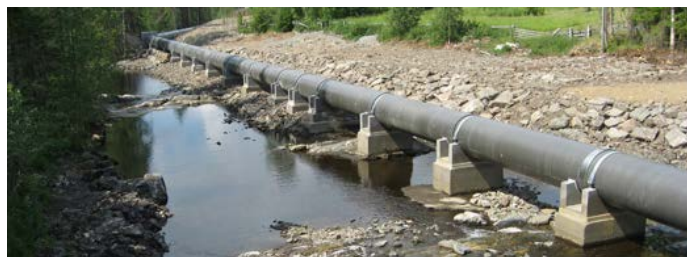
Fig. 4. A typical above ground pipeline
