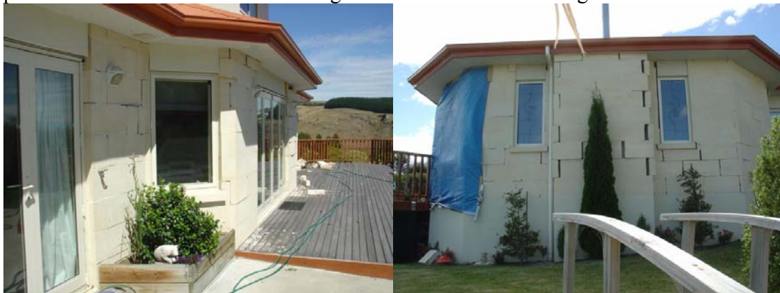
Figure 7 Two storey light steel frame house with Oamaru stone cladding [T Just]
