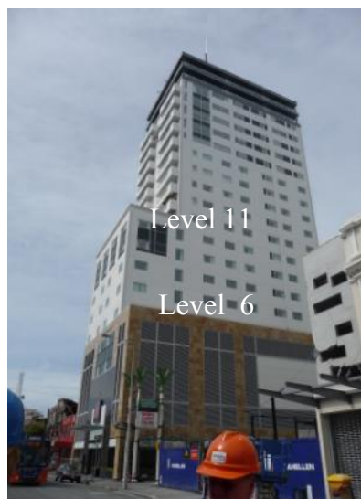
(a) View from North West corner
