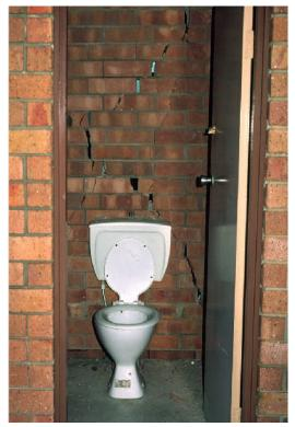
We surmised that the damage could be attributed to the foundations with parts of the city and Hamilton underlain by alluvium hydrauliced from the Hunter River bed to deepen the river channel. Such materials are notorious for adding to earthquake damage by trapping and magnifying the seismic waves and for failing by slumping or liquefaction.
