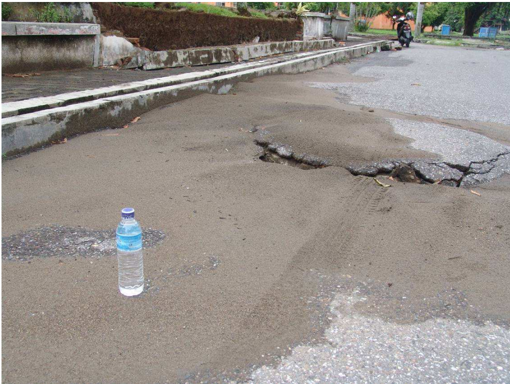
Figure 23 Sand brought to the surface due to liquefaction
