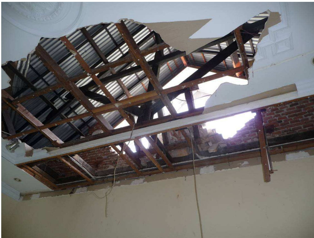
Figure 9 Failed Gable Wall
