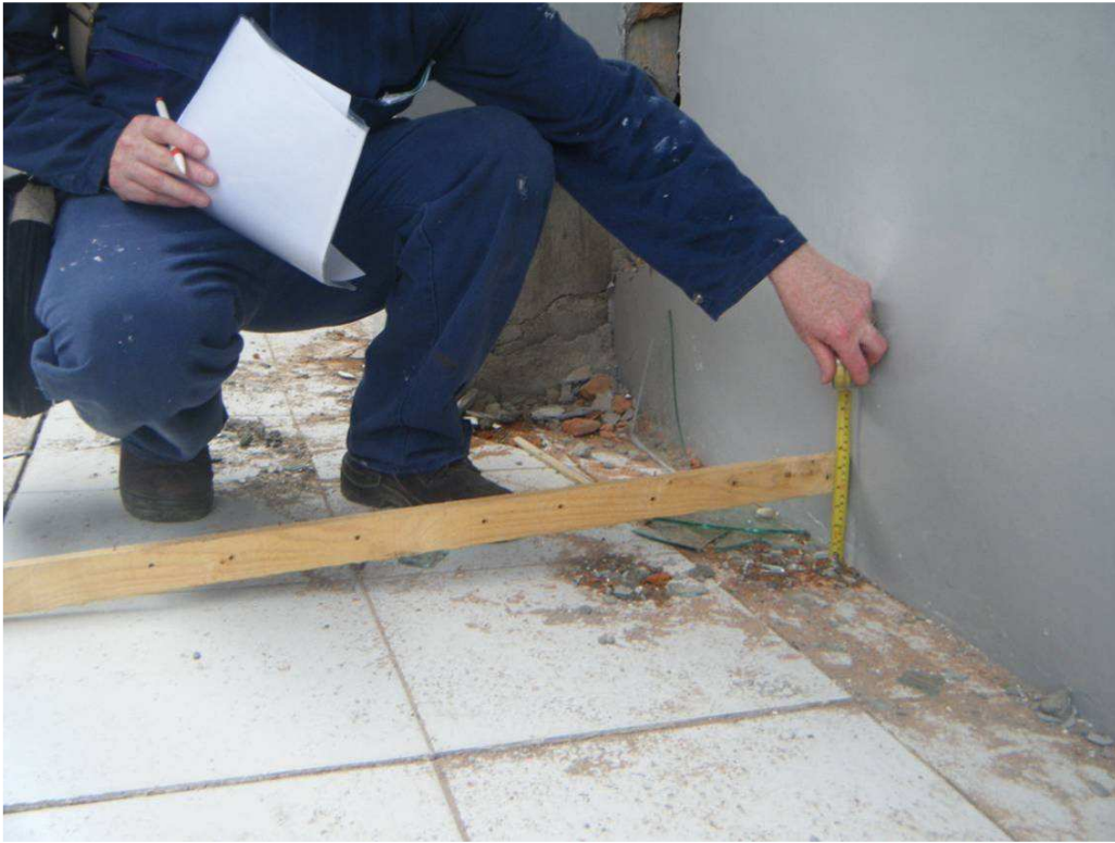
Figure 24 Liquefaction caused heavier buildings to sink
