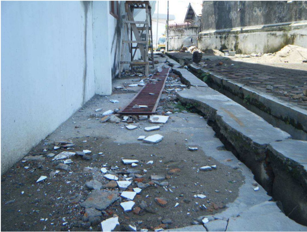
Figure 22 Settlement due to liquefaction (note sand forced up through cracks in concrete)
