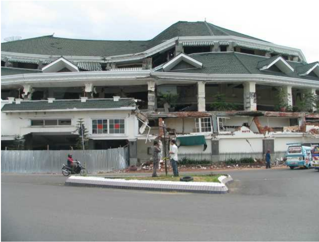
Figure 12 The 6 storey part of this hotel totally collapsed
