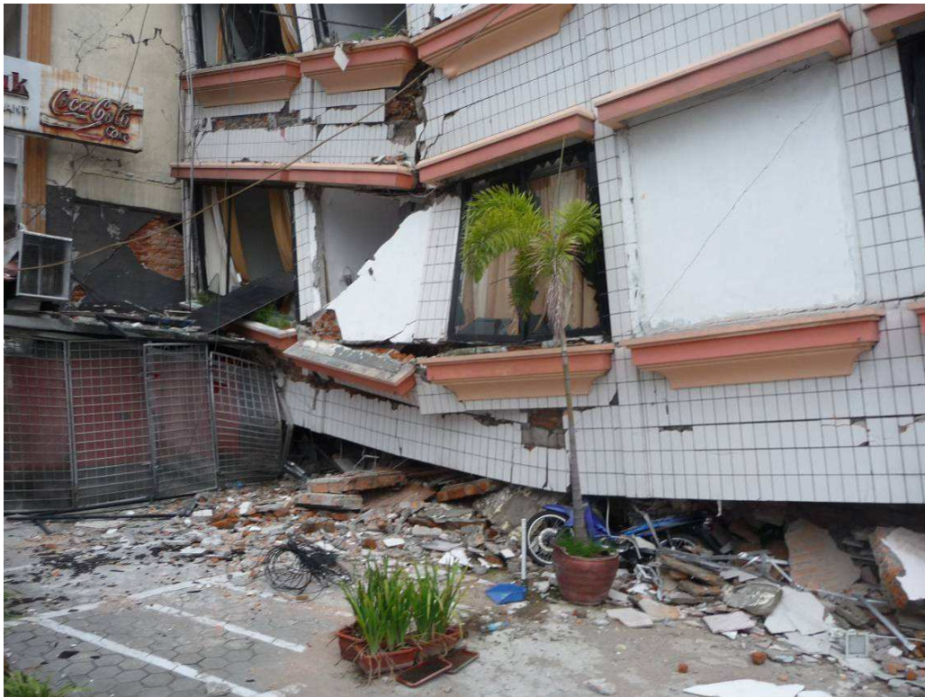
Figure 19 Soft Storey (commercial shop-front) Ground Floor Collapse
