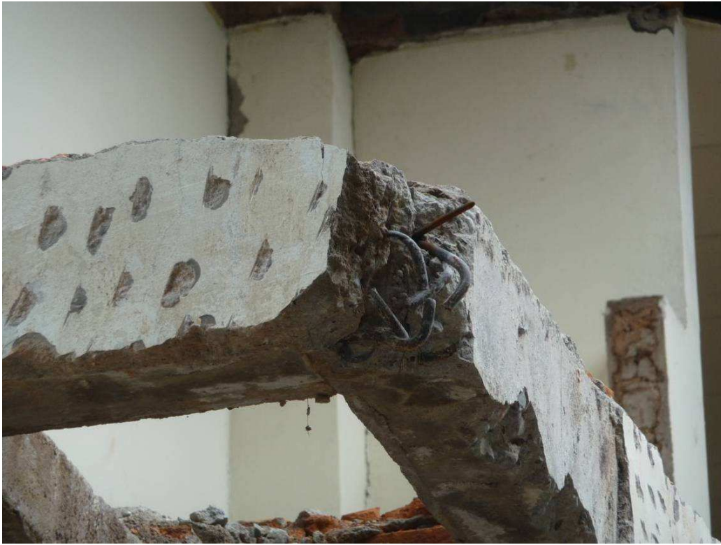
Figure 4 Poor reinforcement detailing
