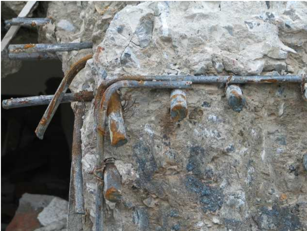
Figure 5 Poor reinforcement detailing
