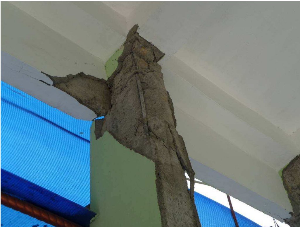
Figure 7 Missing ties in column/joint
