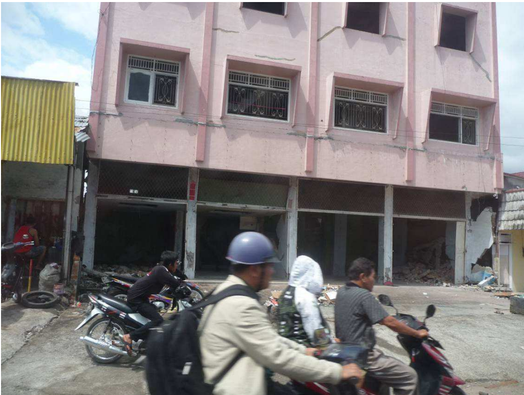
Figure 21 Another soft storey building near collapse
