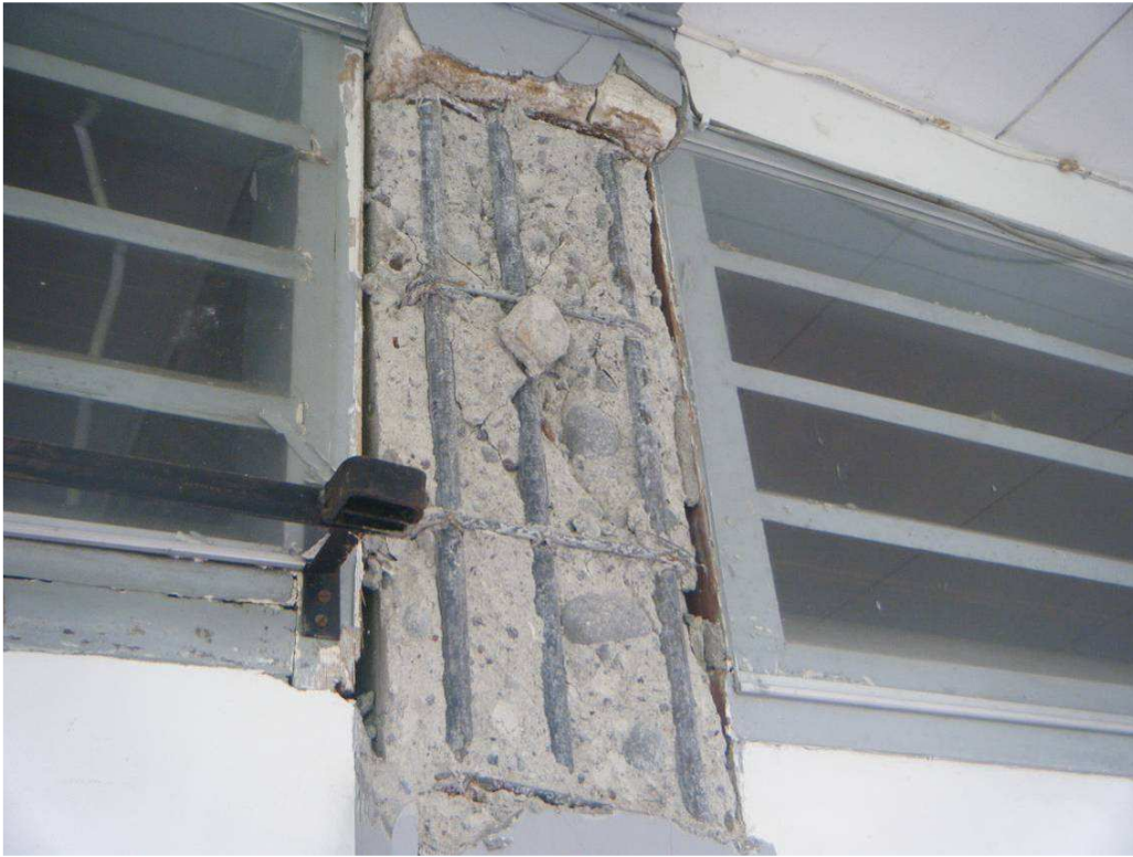
Figure 10 Poor aggregates/concrete
