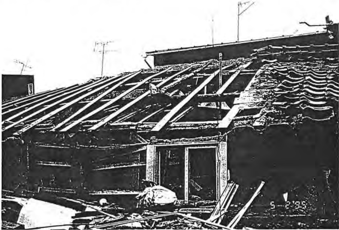
Figure 4 - Tile roof failures
