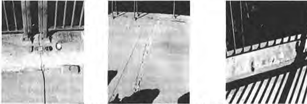
Figure 1, 2 & 3: Showing evident of developing cracks
