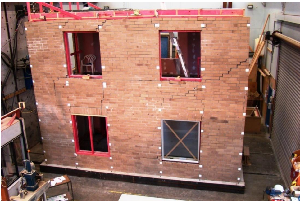
Figure 2 Views of rocking panels – single and two storey specimens
