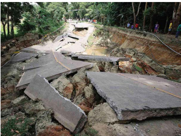
Photo The main concrete road to Buenavista on Bohol seems to have been destroyed by landslide or mass soil movement.
